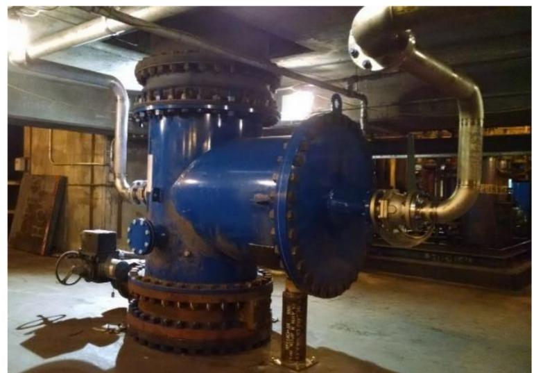
Figure 2. Installed Innovas Ball Trap
